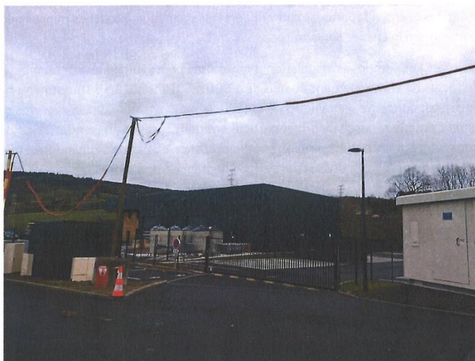
Figure 13 – services techniques – Opportunité 5 - 60 kWc
