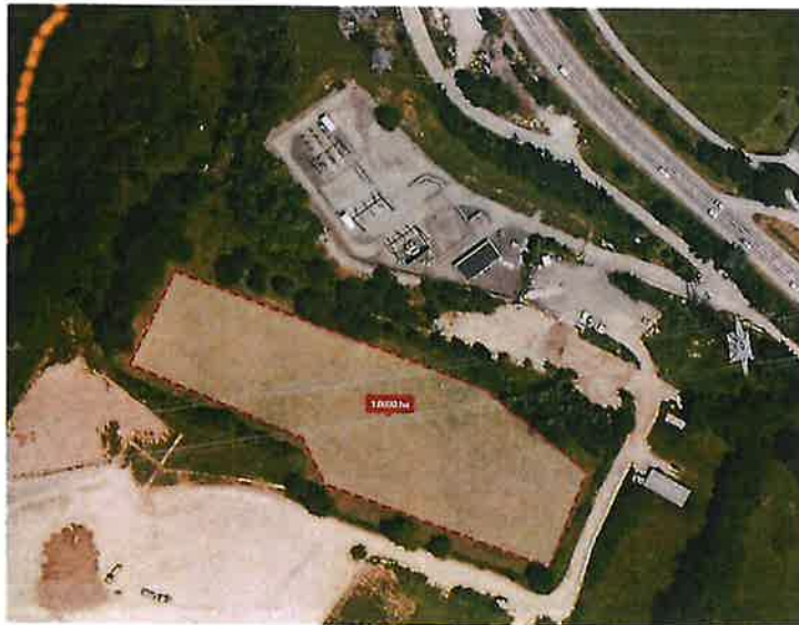
Figure 17 - Opportunité 2 - zone de stockage - 700 kWc
