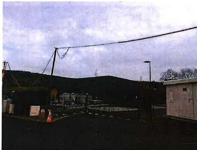
Figure 13 – services techniques – Opportunité 5 - 60 kWc
