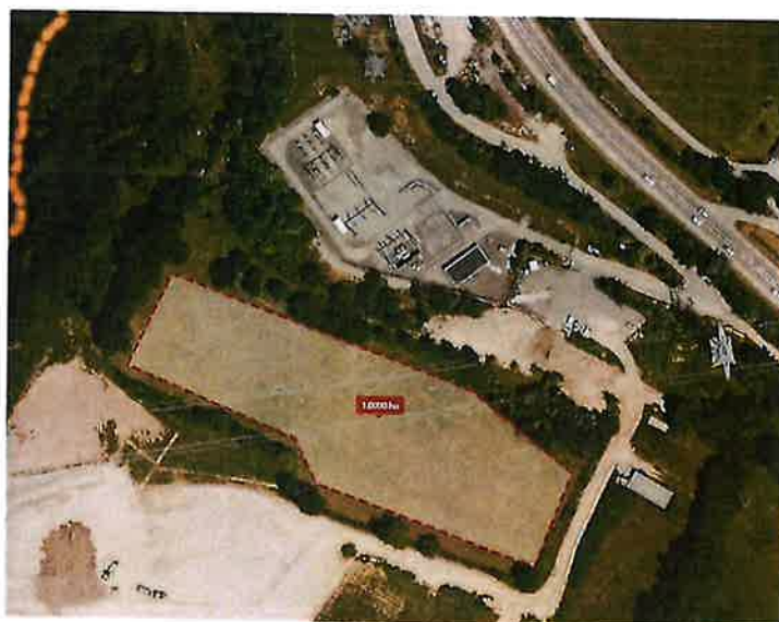
Figure 17 - Opportunité 2 - zone de stockage - 700 kWc
